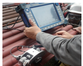
Corrosion Inspection of Boiler Water Wall
